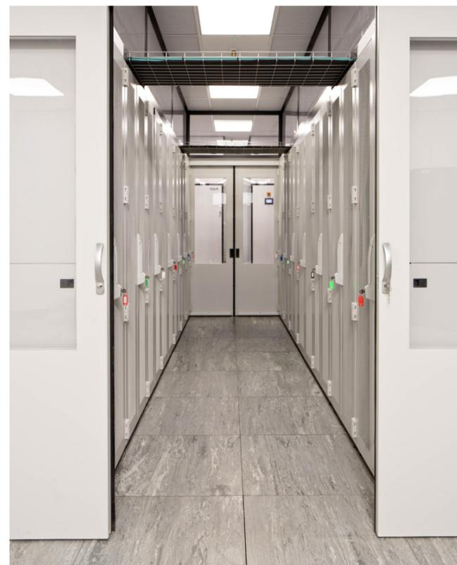
The final **modular data centre** design incorporated 20 cabinets, full power supply infrastructure including generator hook up, hot aisle capture configuration for energy efficiency, Novec Fire suppression and Wagner early particle detection to ensure safety as well as energy efficient air conditioning and UPS systems in an N+1 format and all 19" cabinets included intelligent power distribution.
